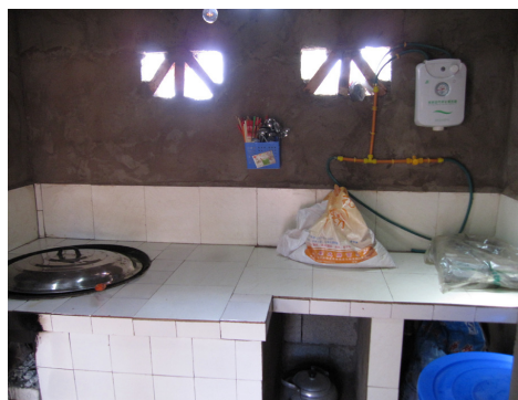
Construction of bio-gas stove in Meigu County, Sichuan Province
